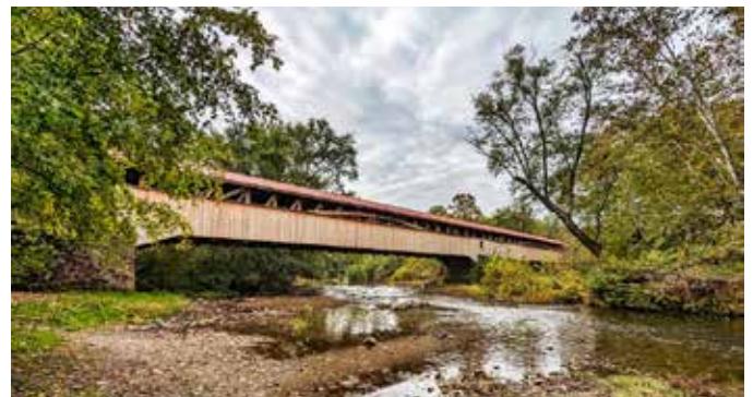
Pomeroy Acedemia Covered Bridge.
